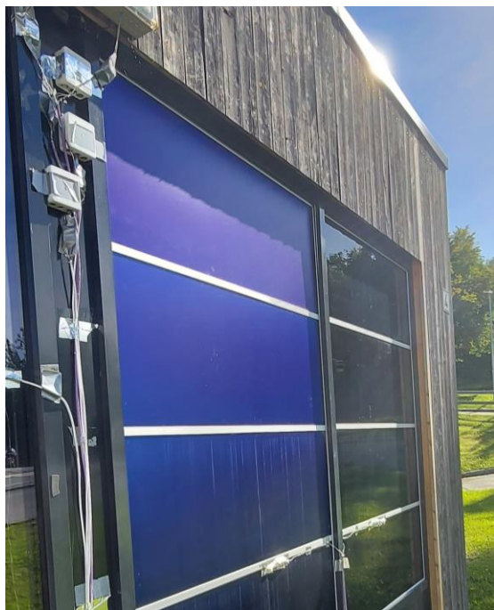
Fig. 3. A shadow formed by the building design at the top panels, noticeable in the warmer part of the year
